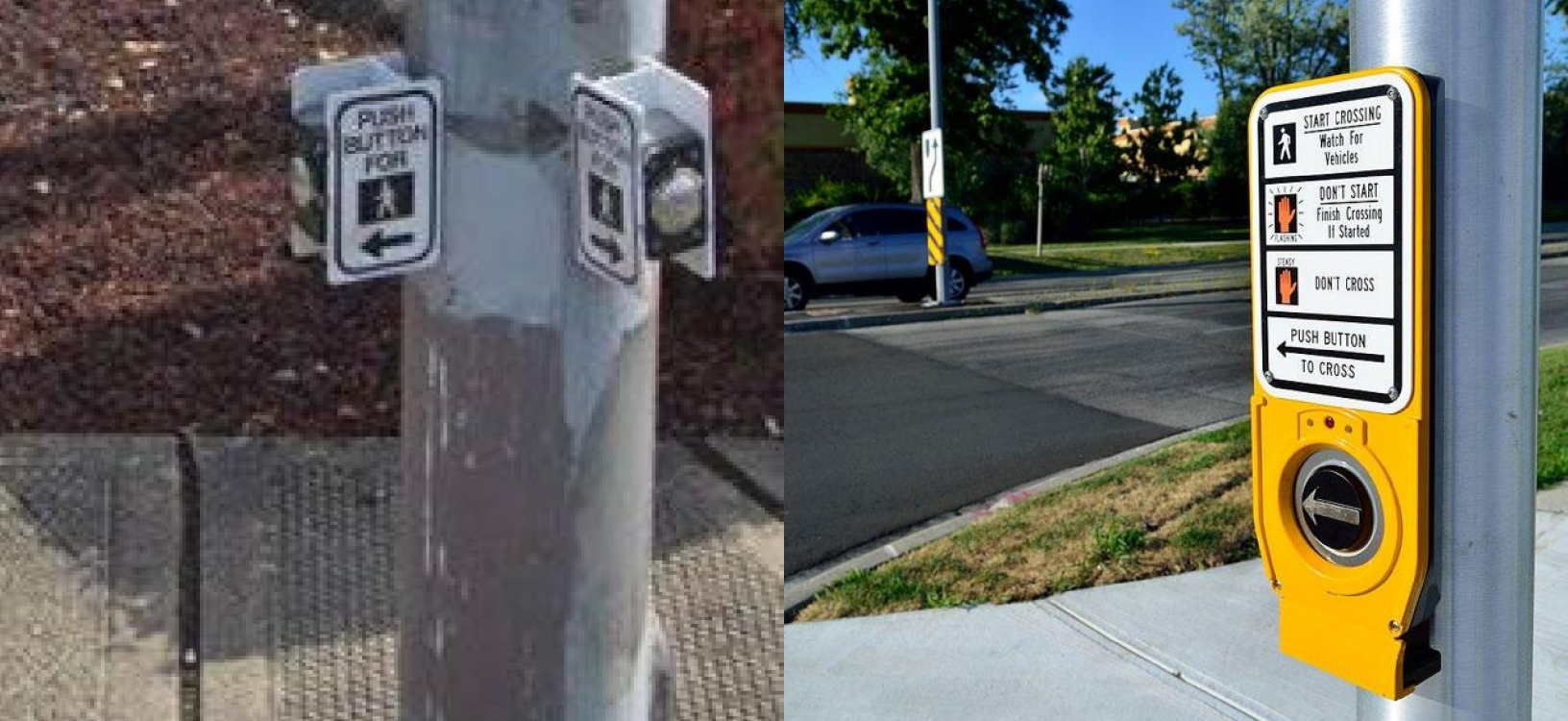
Figure 2-10 “H-style” (left) and APS-style pedestrian pushbutton (right)
